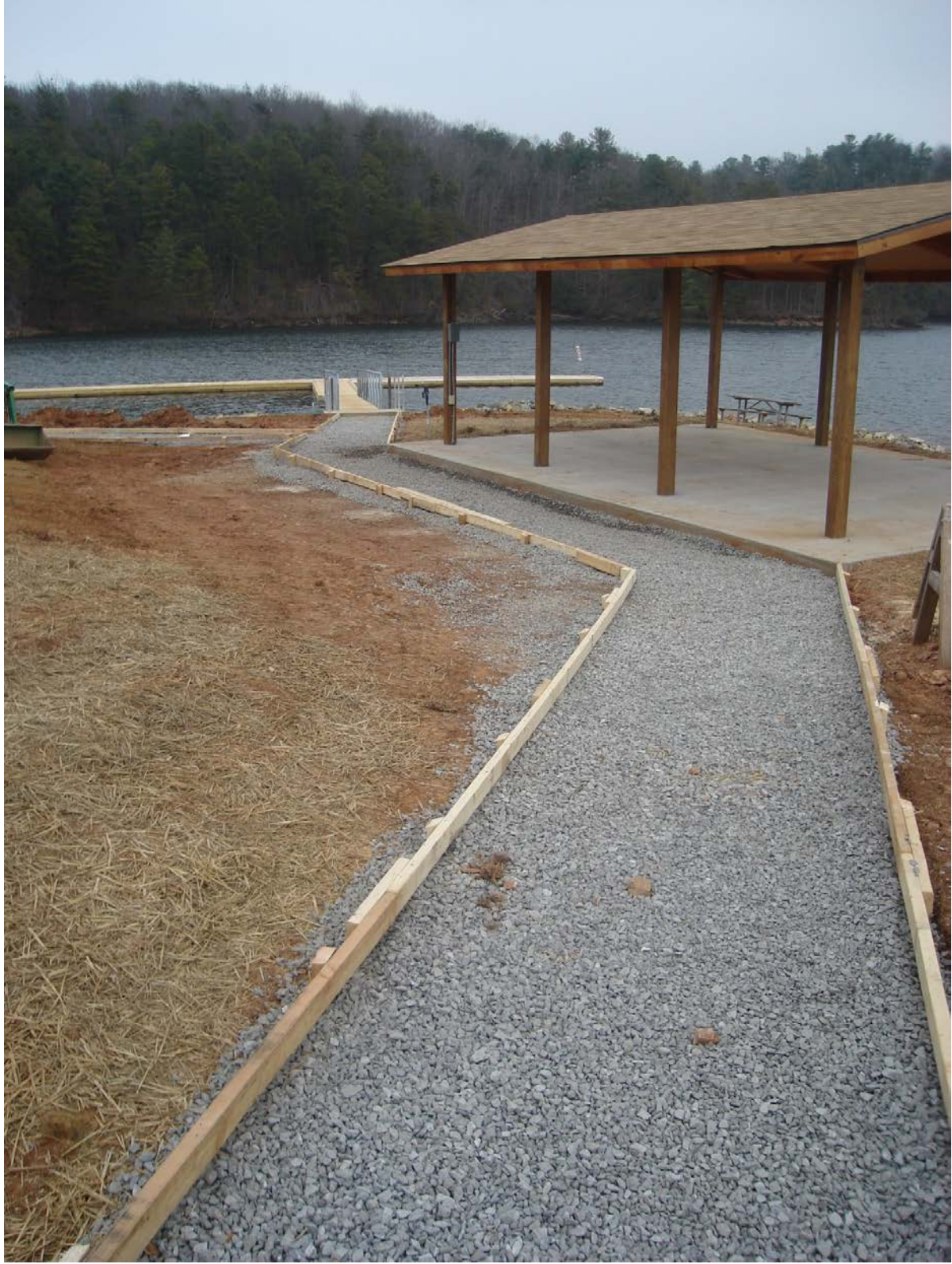
Forming ADA Sidewalks for Twin Ridge Fishing Tournament Central Handshake Partnership
